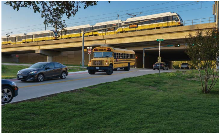
The intersection at Cistercian Rd. now features DART trains and a traffic signal.
