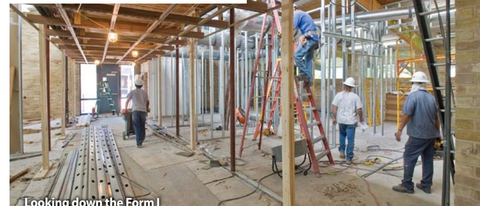
Looking down the Form I hallway towards the Upper School.
